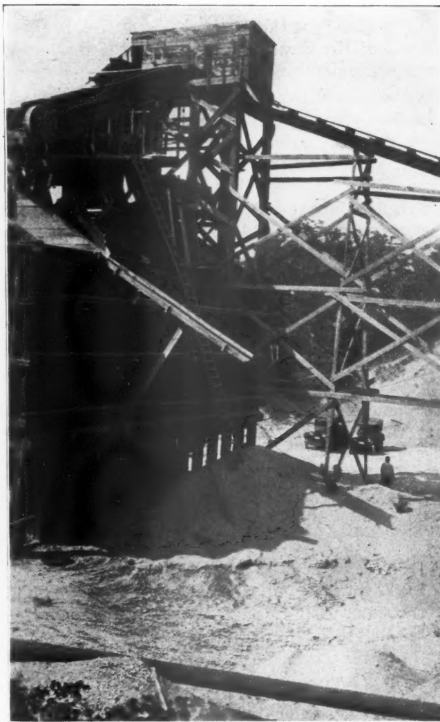
Sizing Screens with Storage Bins Below
